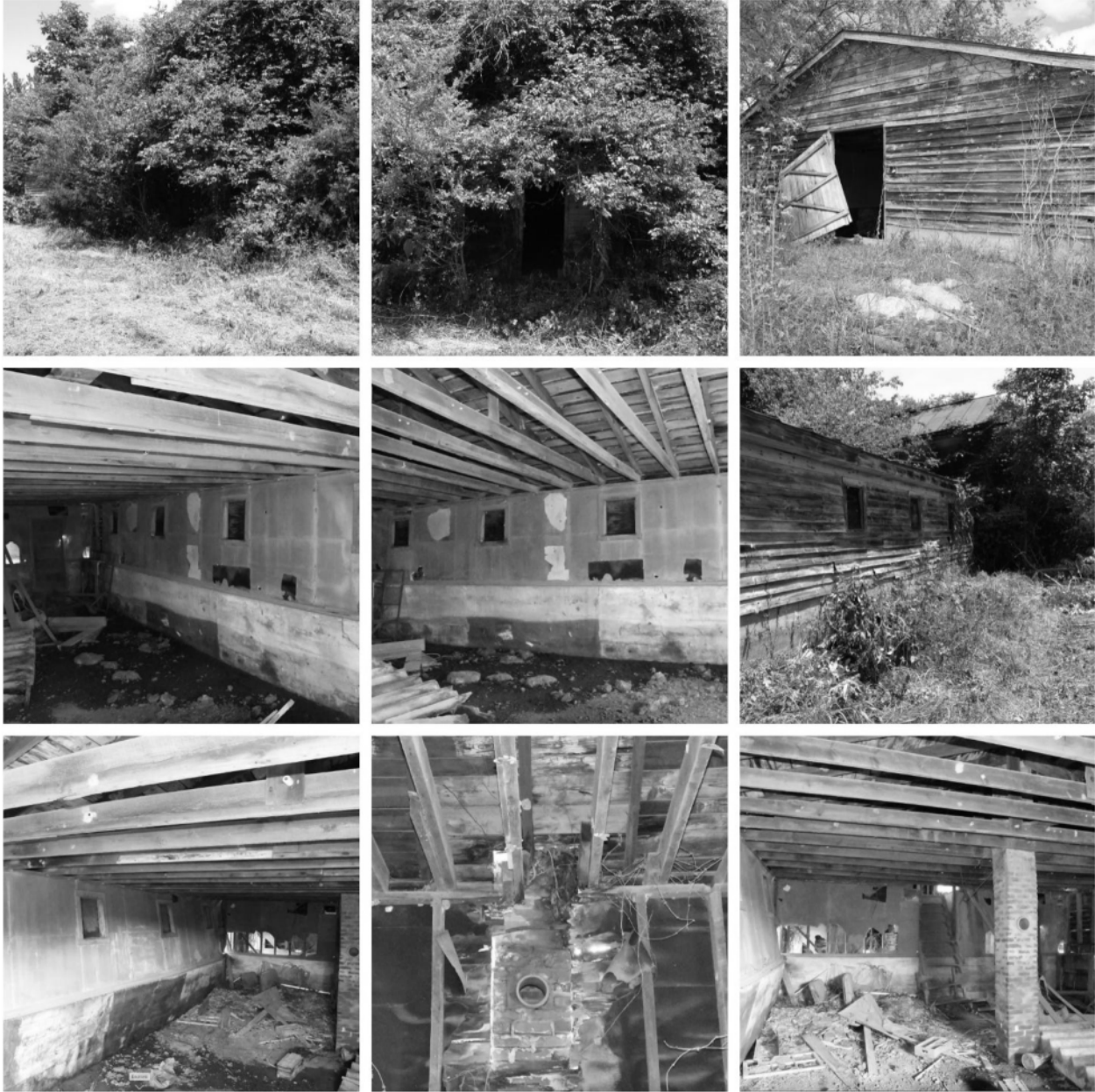
Some of the "Before" photos
